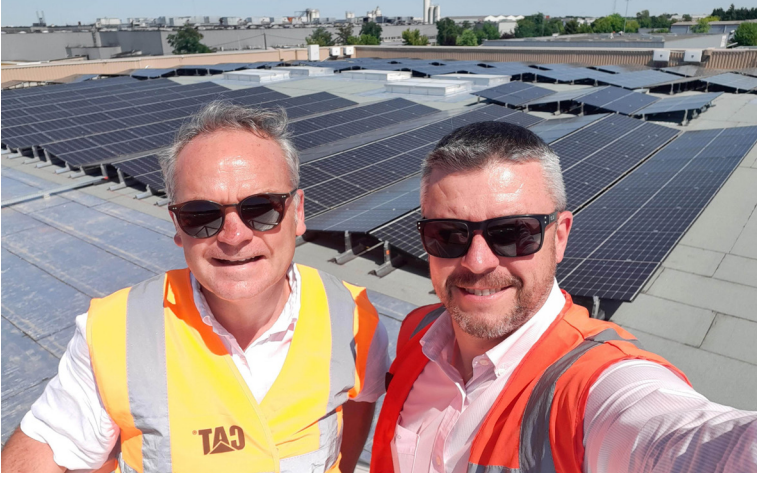
Commissioning of the solar power plant at the new GCS site in France.
